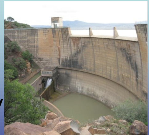
Lubisi Dam (at present)
